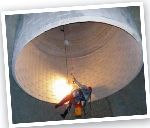
Maintenance of CVF , Czech Republic. A mountaineer is doing the inspection in an unusual way. Normally the inspection is carried out visually from the manhole or by erecting a scaffolding.
