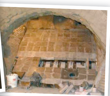
Precast slope in the smoke chamber, Czech Republic
