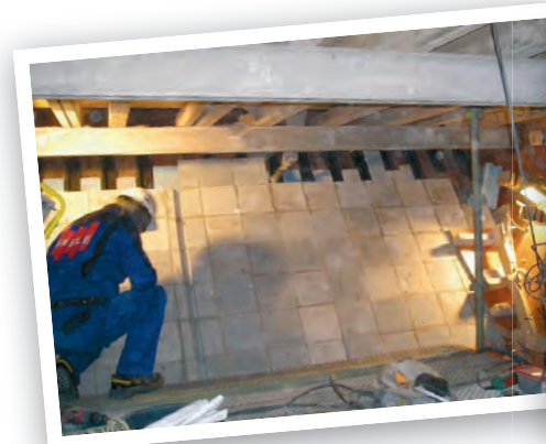
Precast pyro chamber, Norway
