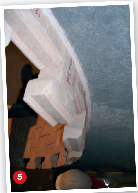
Ready to close the top ring of elements on the suspension brackets.
