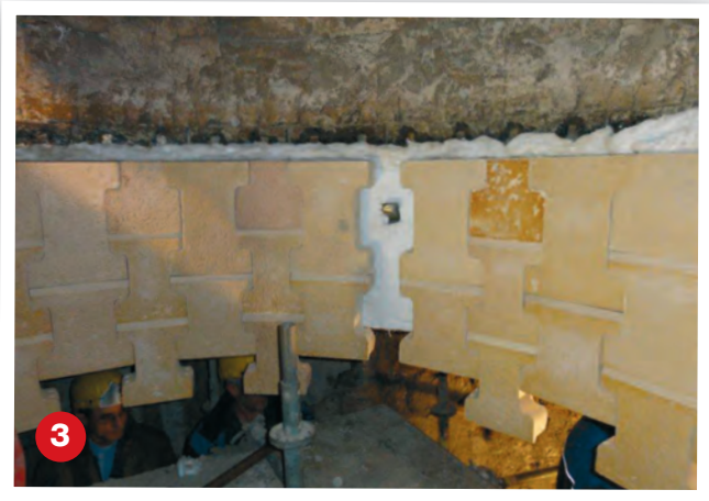
Ready to close the top ring of elements on the suspension brackets.
