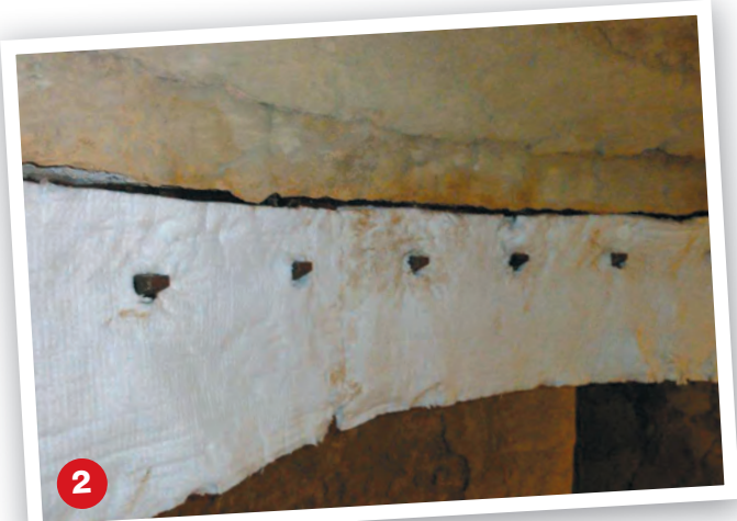
Ceramic fibre blanket is installed - to allow for thermal expansion.
