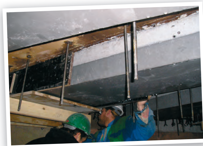
Casting the cyclone roof, Czech Republic
