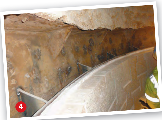
The top ring of precast elements are installed.
