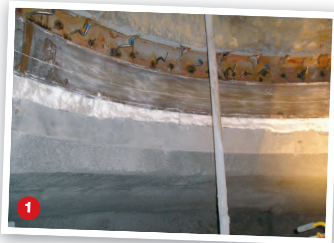
A steel ring is welded into the roof of the cyclone.
