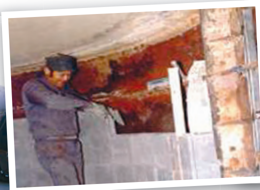
Precast walls and cones, Mexico
